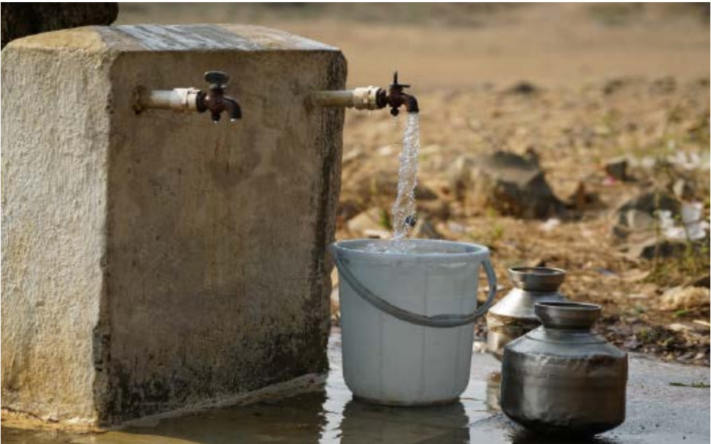
----- Figure 3C.12: Standposts in village
