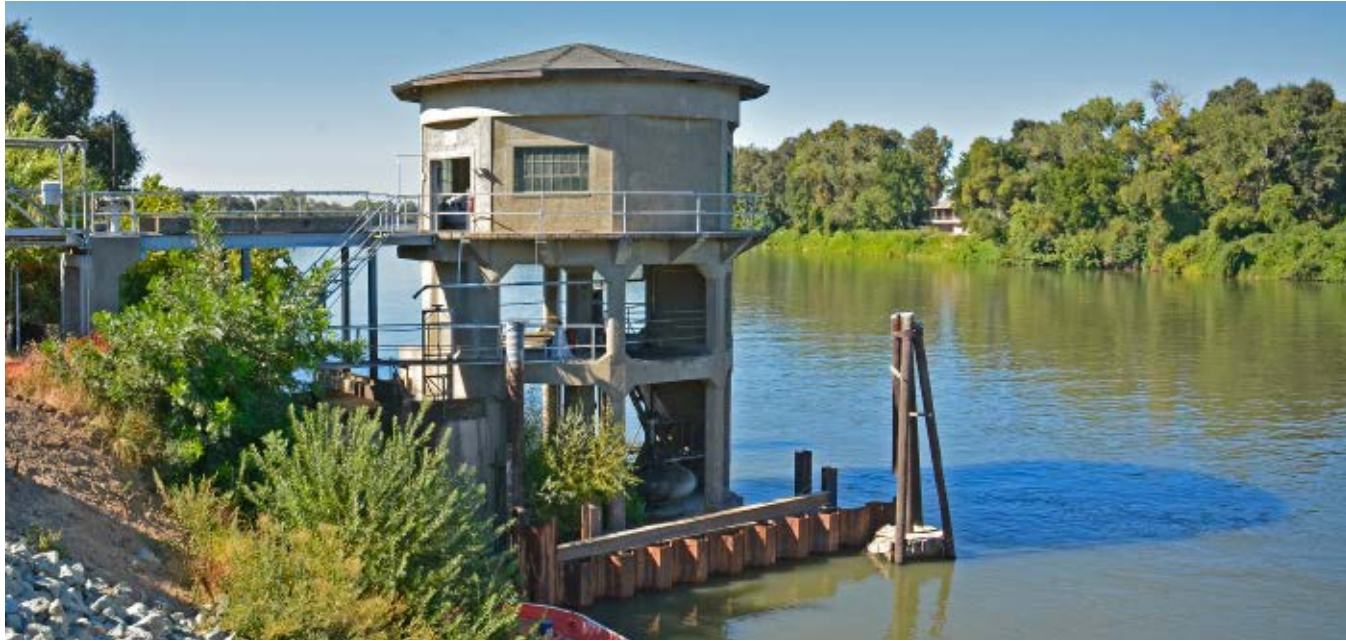
Picture 2.2: River intake structure
