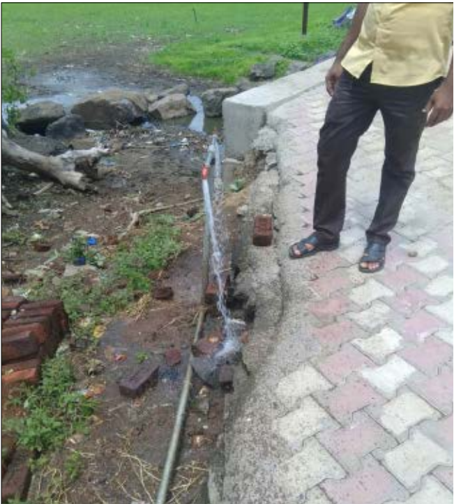
Figure 3C.9: Distribution network laid on ground
